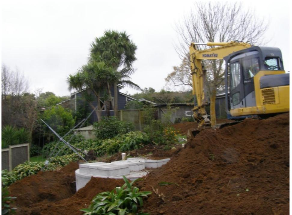
The Airogreen Wastewater System is a single unit tank. It can be buried without problem and only 50mm of the risers & lids need to be above ground to allow the system to breathe in the air used in the process & to prevent ground water ingress
